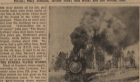
Engine No. 2 in the place of a mill, with a mill of supplies as seen in Camp Carson.
