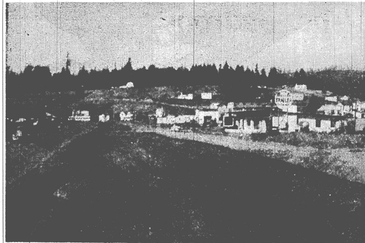
When completed, this will be a four-lane highway.
