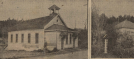
Old Garfield school in center of Freshwater teachers' quarters of the days of Washington.
