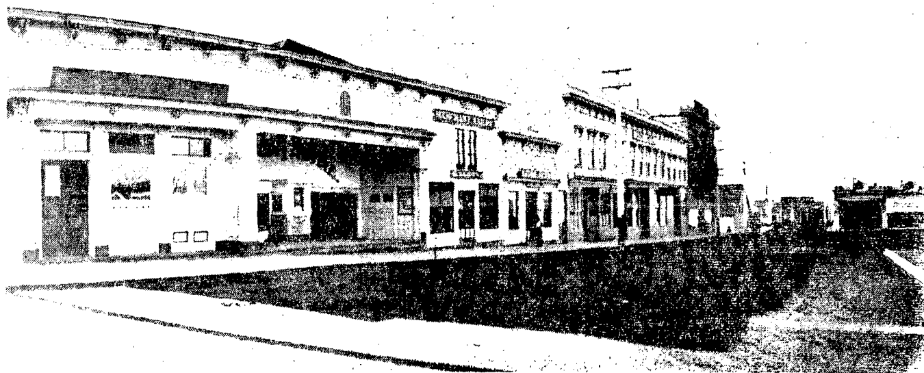
Along 8th street, showing the old Post Office. About 1913.
