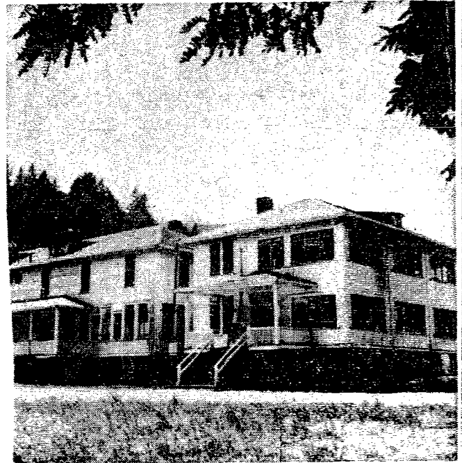
HOOPA — The future of the Hoopa Branch of the Humboldt County Library looks uncertain. The old building was originally built for a boys dorm and later became a school building. Its last usage was as housing for teachers at the Klamath-Trinity Unified schools. It is now condemned and abandoned except for the library. It is to be razed in the near future.
