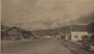
Looking north on Highway 99--Orick's "main street" with railroad track bridge and new concrete bridge in distance.
