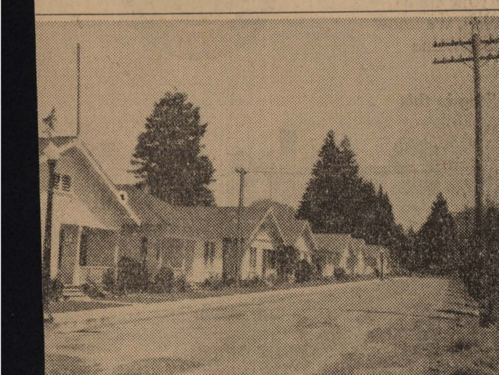
oad avenue, Scotia, offers a decided contrast to most streets along main line tracks.
