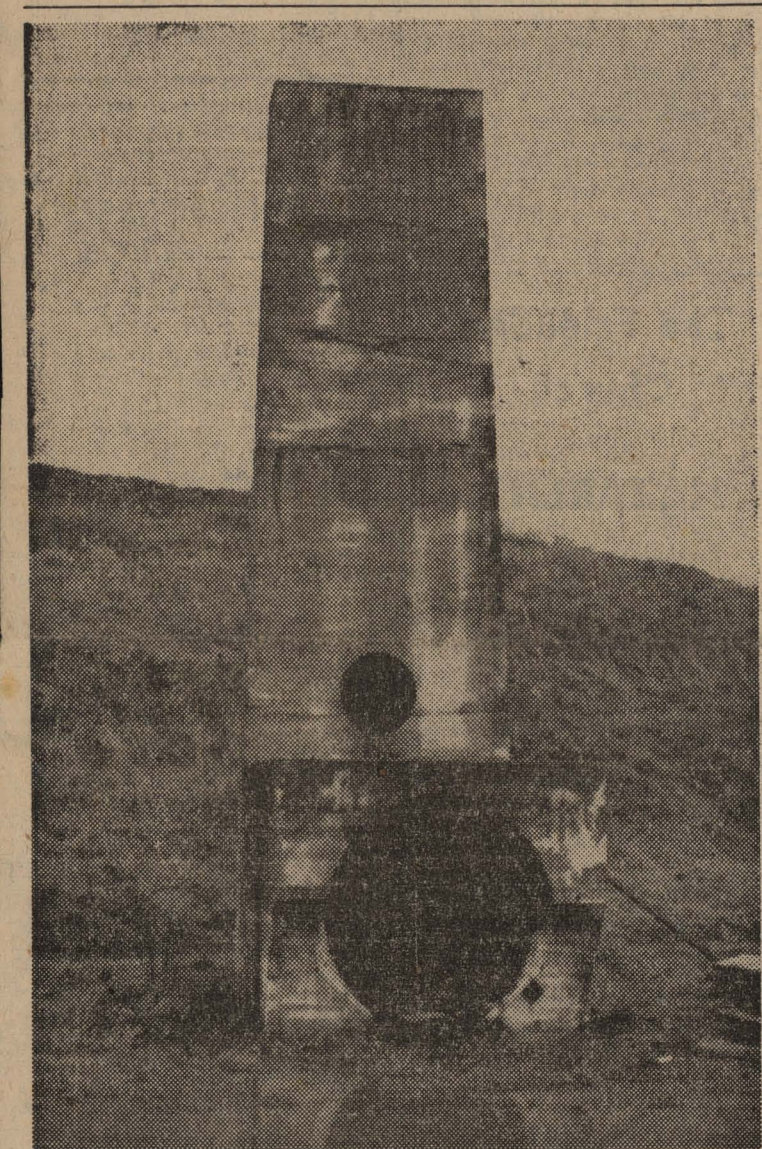
Old whaling boiler stands stark
